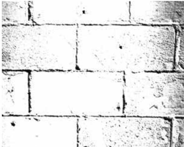
Figure 10a. An example of a deteriorating block wall.
